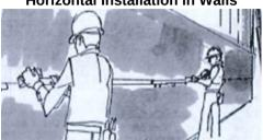
Snap a line across the entire wall length to establish a straight edge. Measure the length to be applied from corner to corner, allowing an additional amount of overlapping. Starting at the bottom of the wall, overlap the foundation approximately 3", keeping the top edge parallel to the snap line. Wrap around the corner and staple or tape in place. Install the next length parallel to the first length, overlapping the first layer 2".
