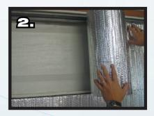
Remove the release liner from the tape and firmly press the reflective insulation against the adhesive, working from side to side or top to bottom. Trim any excess insulation.
