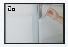
Measure and cut each roll of insulation to fit over the mounted strips of doublesided tape. Test fit each piece to ensure proper sizing for each panel.
